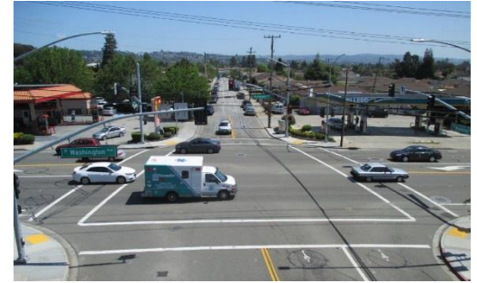
Signal at Washington Monterey funded by DFSI
