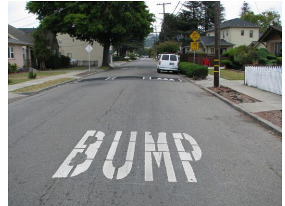
Durant Ave Speed hump installed under Traffic Calming program
